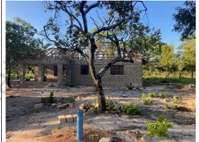
Photo 39: Replacement house under construction
