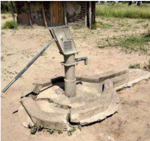
Figure 19: Sikuka Handpump / Borehole
