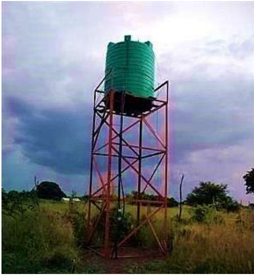
Figure 21: Sikuka Water Tank and Stand - Muyabalo Community Club
