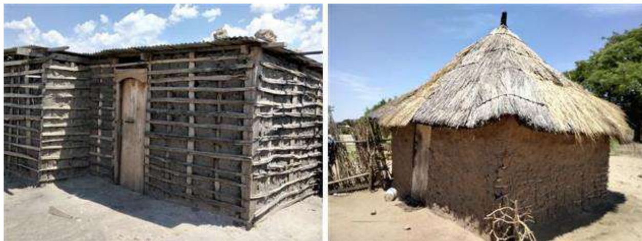
Figure 11: Typical Residential Structures
