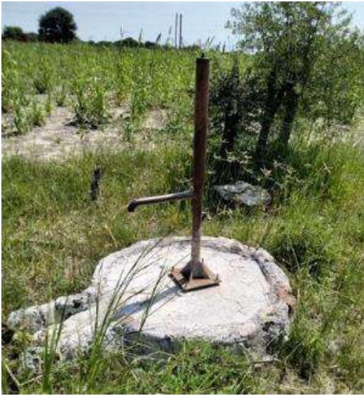
Figure 20: Sikuka Handpump / Borehole
